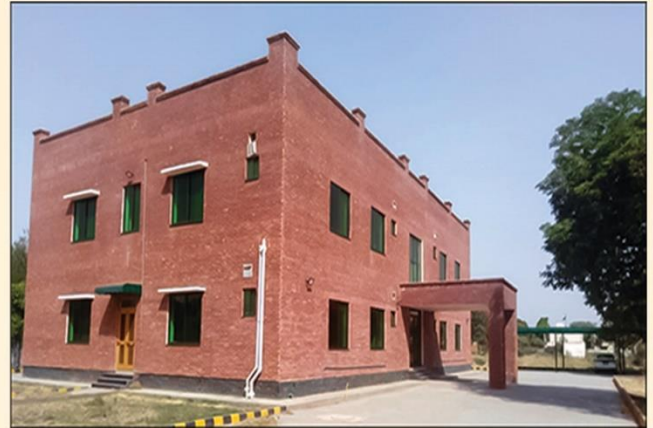
Construction of Double Storey Barrack for Ladies Staff
