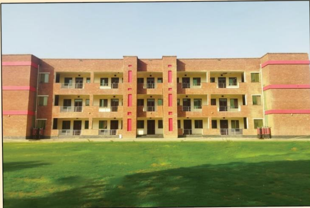
Construction of Triple Storey Living Accommodation for ASF Personnel
