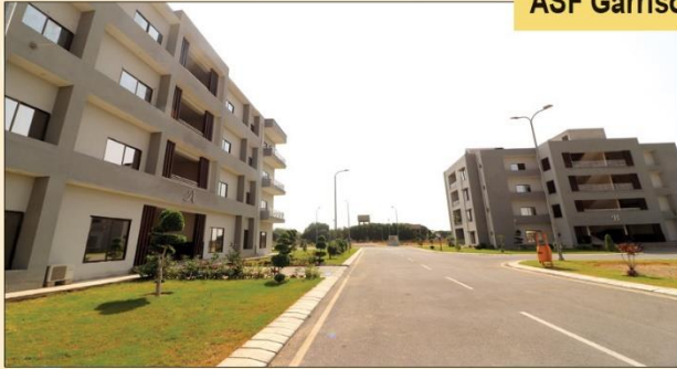
Construction of MOQs.
