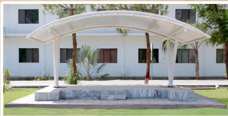
Installation of Tensile Membrane Shade Football Ground
