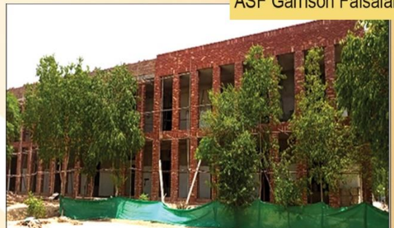
Construction of Double Storey Barrack
