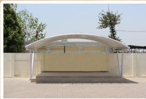
Installation of Tensile Membrane
