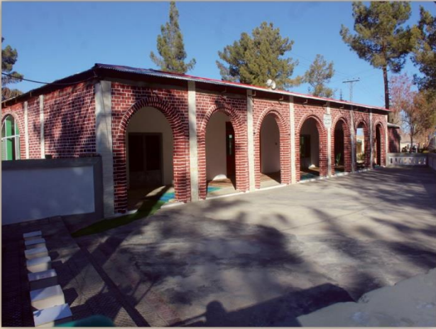
Construction of Unit Mosque
