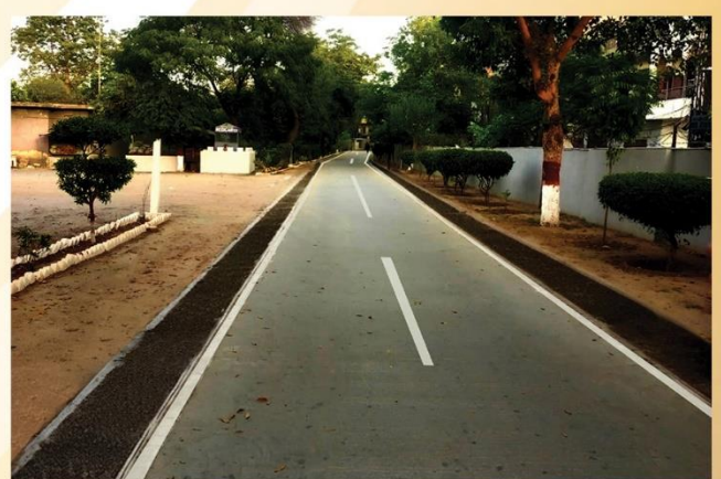
Construction of PCC Road (50 Feet)
