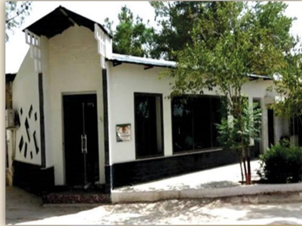
Construction of Unit Welfare Canteen
