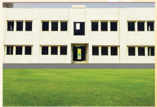
Construction of Girls Block of ASF Public School
