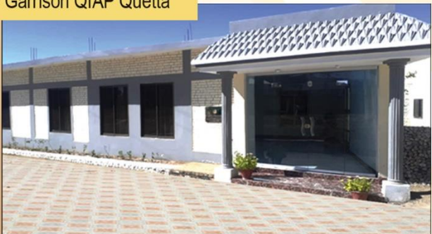
Construction of Officers Guest Rooms alongwith allied facilities
