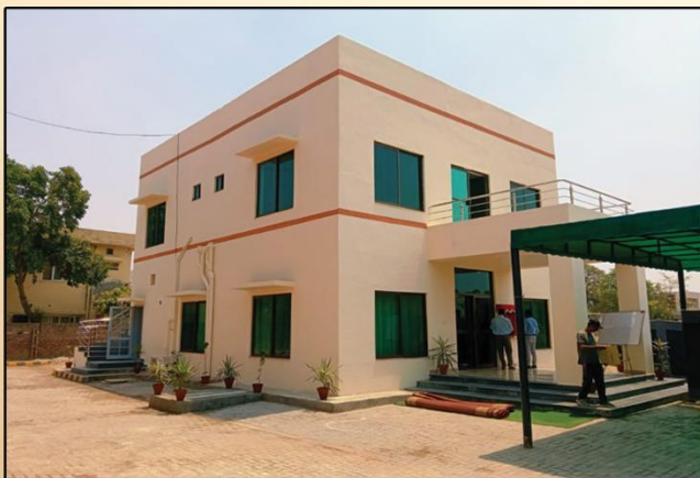
Construction of New Ladies Mess and Recreation Hall
