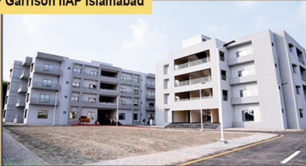
Construction of MOQs.
