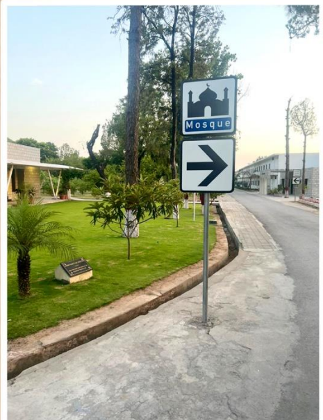
Installation of Sign Boards and Traffic
