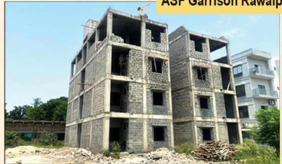
Construction of Junior Staff Apartments
