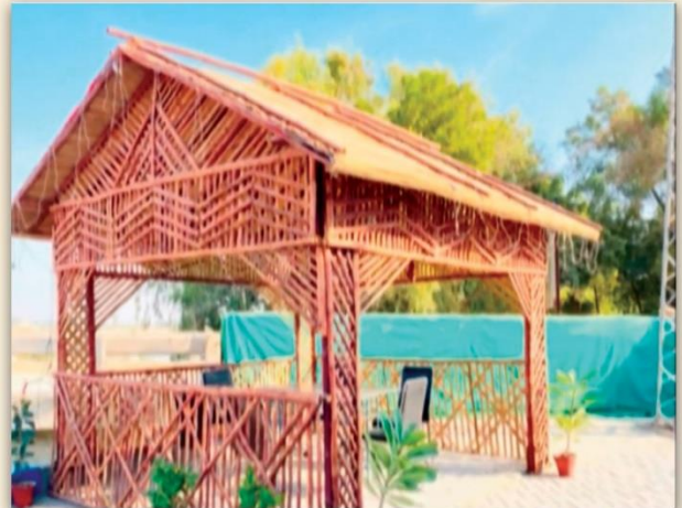
Construction of Bamboo Hut
